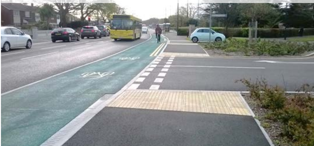
Figure 10.17: No setback crossing with design priority,– Bournemouth
