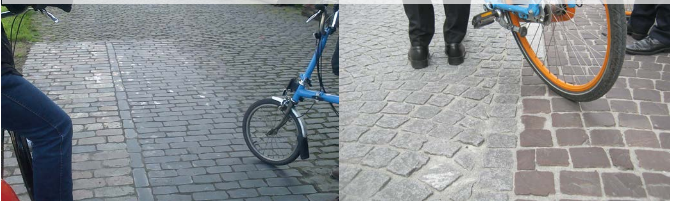
Figure 7.9: Trial site in Bristol to provide smoother surface, and similar application in Bruges with setts in a different colour from the adjacent traffic lane.
