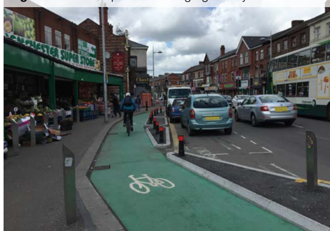
Figure 1.10: Example of kerb-segregated cycle track
