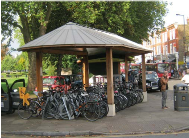
Figure 11.10: Small cycle hub at Ealing Broadway offering CCTV secure parking and cycle hire
