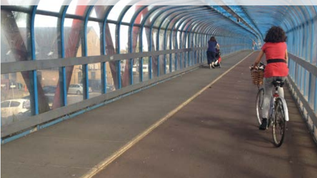
Figure 10.50: Covered pedestrian/cycle bridge across railway tracks, Cambridge
