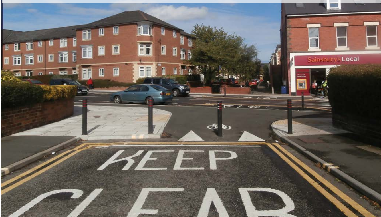
Figure 8.5: Cycle route crossing a footway, Newcastle
