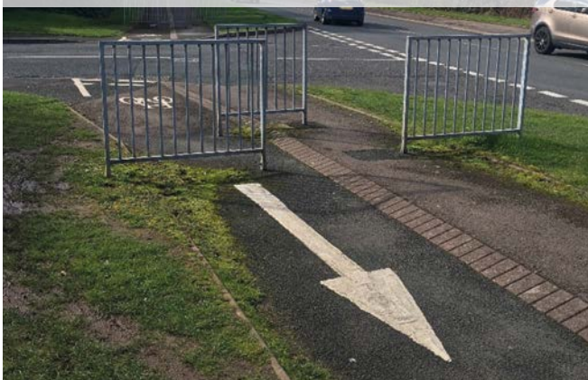
Figure 14.3: Poor quality provision for cycling in a housing development – no priority at side road, compounded by barriers
