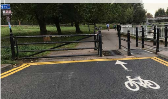
Figure 8.4: Cattle grid access control, Cambridge
