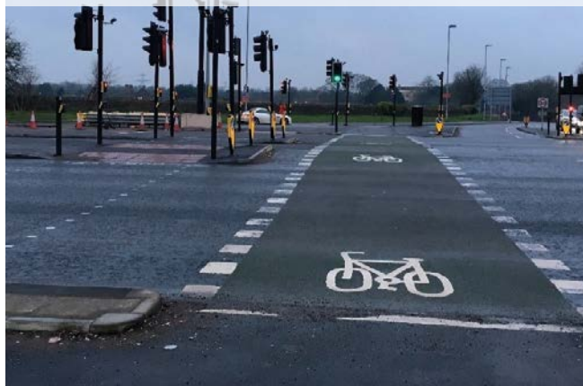
Figure 10.9: Single-stage straight-over cycle crossing next to multi-stage staggered pedestrian crossing, South Gloucestershire
